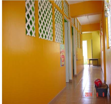
Non Pariel Pre-school After Refurbishment
